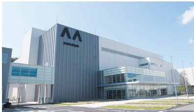
Fukusaki Factory (Japan) Production volume: 110 million units
