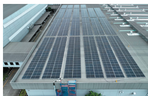
Solar panels on the roof of the new factory production building at Fukusaki Factory
