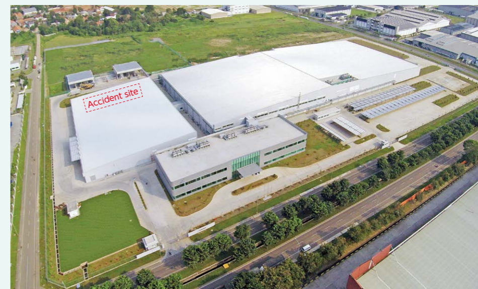
Aerial photo of new Indonesian head office building and cosmetics manufacturing plant (Factory 1) (Feb. 2015)
